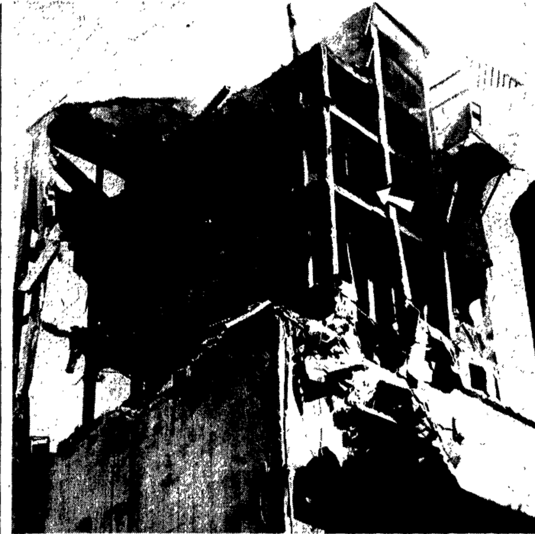
TRAPPED 80 FEET above the ground on a beam amid wreckage of the Saskatchewan Pool elevator at Port Arthur after Tuesday's explosion is a workman, indicated by arrow. Men trapped here were rescued by Pte. Bruce Cudmore, Toronto, who crossed from the structure, right, on a rope shot by a naval rope-gun by tars of H.M.C.S. Griffon
